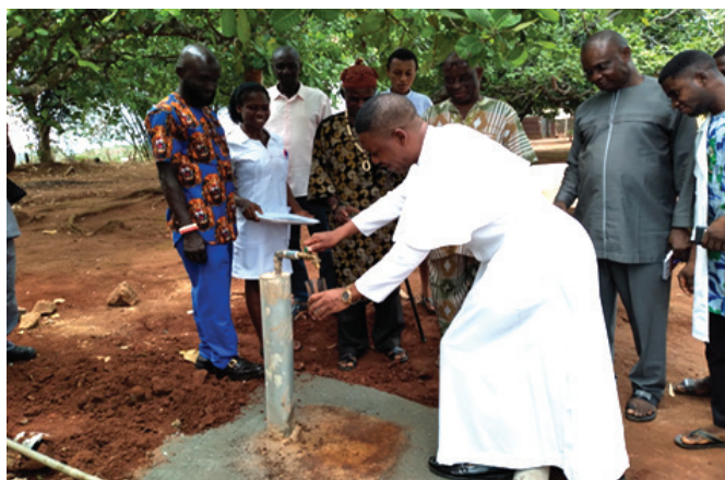
Commissioning one of the boreholes in Nigeria
