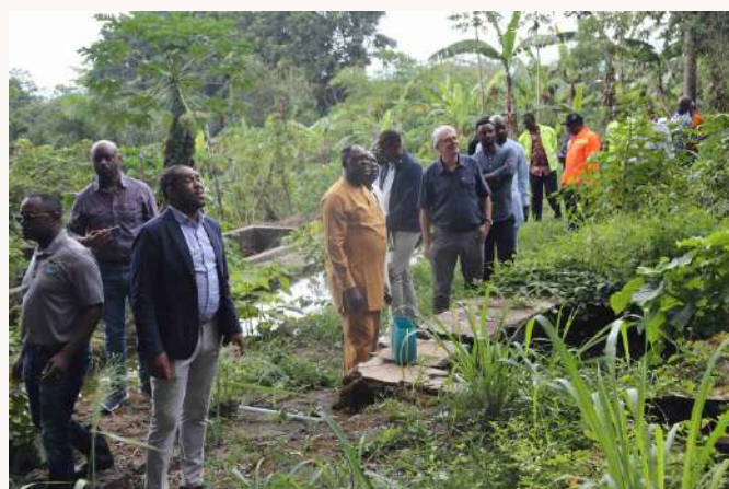
Assessment of the construction site.
